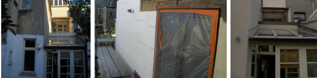
Figure 2: Case study Antwerp: detail of rear insulation (first, intermediate and final steps). Source: PHP, arch. G. Camerlinck; Photo: E. Mlecnik
